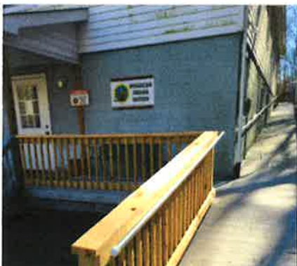
New concrete ramp along backside of Tribal Hall.
